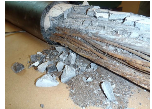
Post-Tensioning Grout (SS 938)
