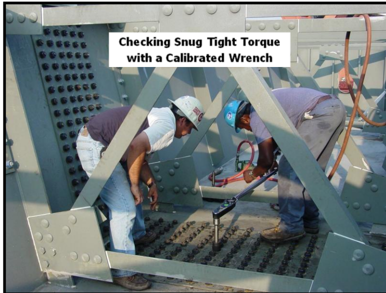
Figure 8 – CEIs Performing Verification Tests for Snug Tightness
