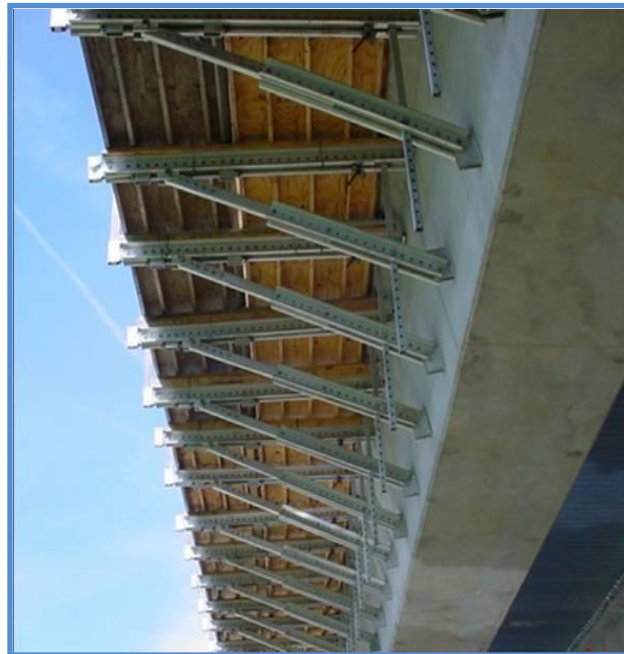
Figure 19 - Form Overhang Brackets
