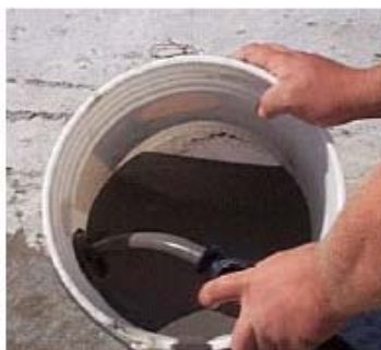
Figure 13, Discharging good grout from vent pipe
