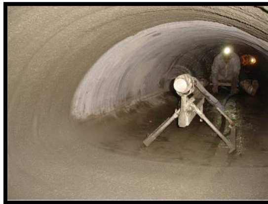
Centrifugally Cast Concrete Pipe Liner
