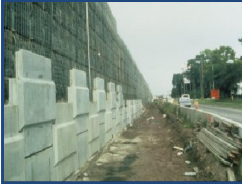
Figure 15-2: Temporary and Permanent Wall Facings
