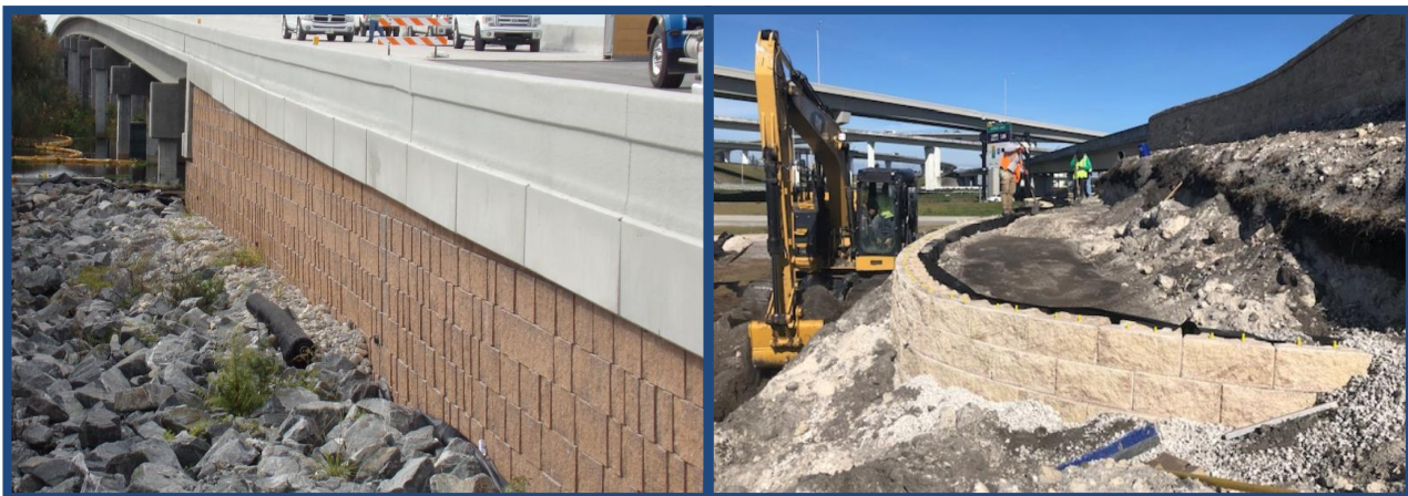
Figure 6-2: Segmental Block Walls
