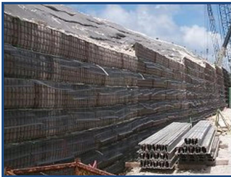
Figure 15-1: Temporary Facing during Phased Construction
