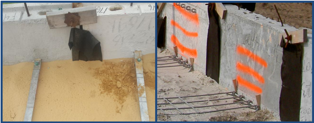
Figure 7-7: Reinforcement Connections
