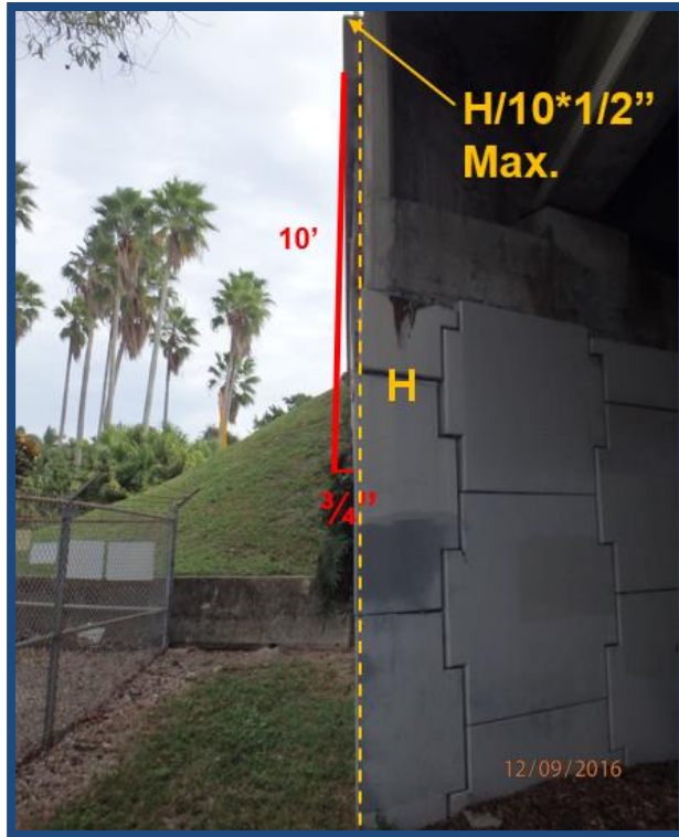
Figure 20-1: Vertical Alignment Requirements for Permanent Concrete Panel Walls
