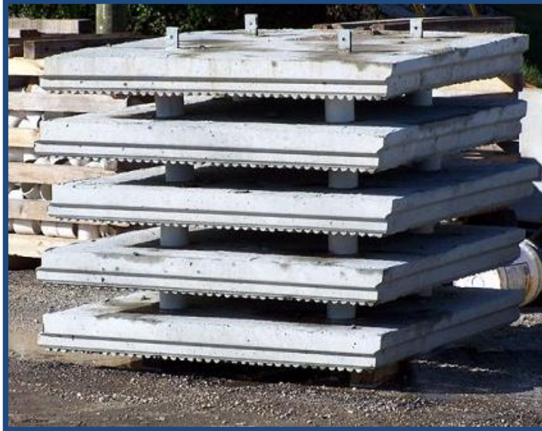
Figure 6-8: Proper Panel Storage
