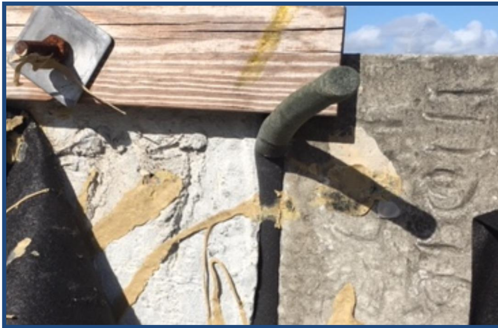
Figure 9-2: Joint Compressible Free Draining Seal to Prevent Vegetation Growth
