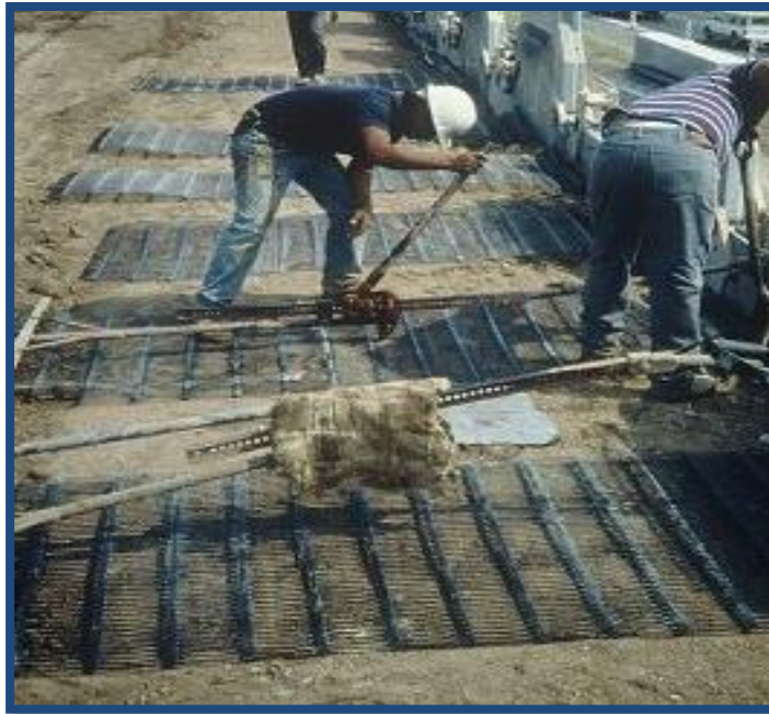
Figure 17-7: Tightening Polymer Reinforcement
