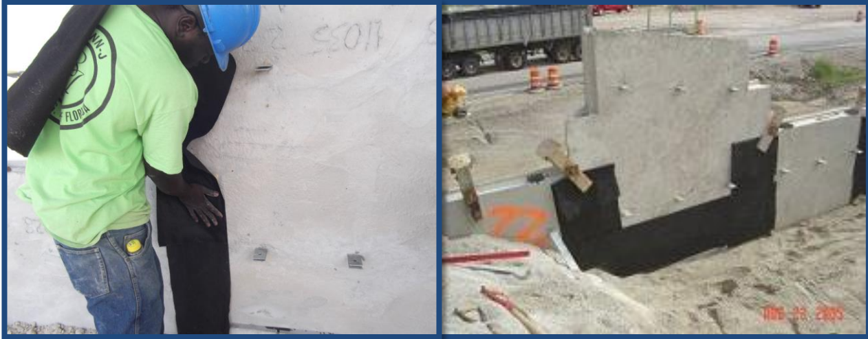
Figure 8-1: Filter Fabric Installation
