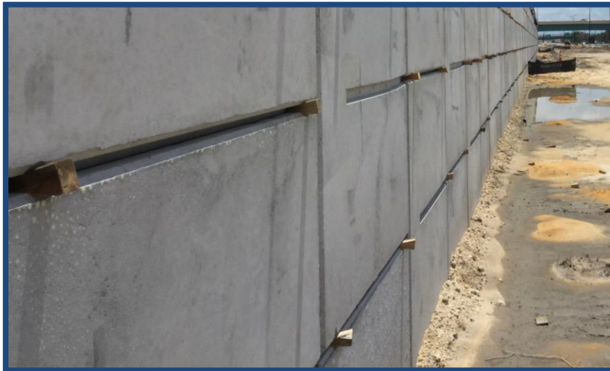
Figure 6-7: Wooden Wedges
