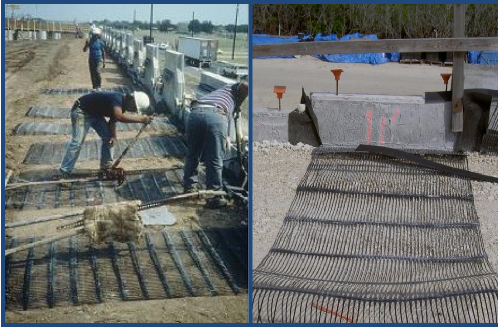
Figure 7-3: Geosynthetic Reinforcement (Extensible)
