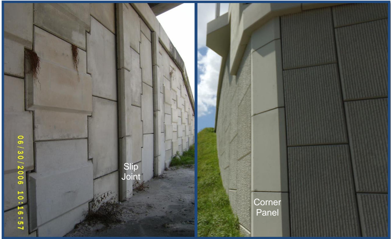
Figure 6-6: Slip Joints and Corner Panels
