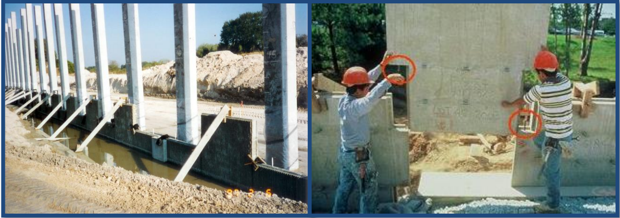
Figure 6-4: Placing and Bracing Panels
