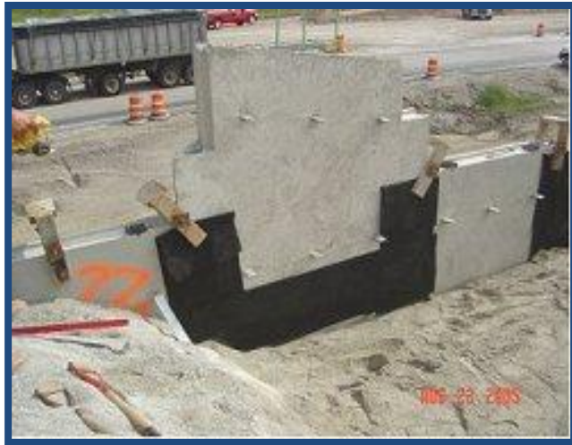
Figure 17-4: Attach Filter Fabric
