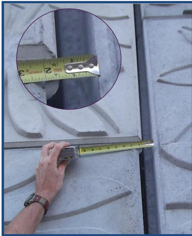
Figure 20-2: Joint Opening Measurement
