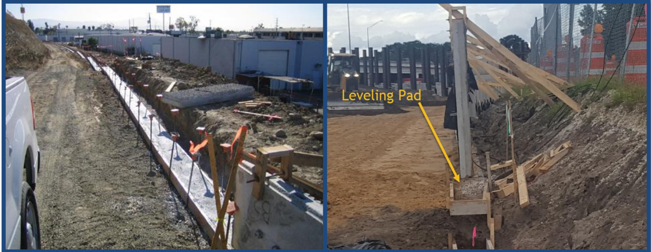
Figure 5-1: Proper Leveling Pad
