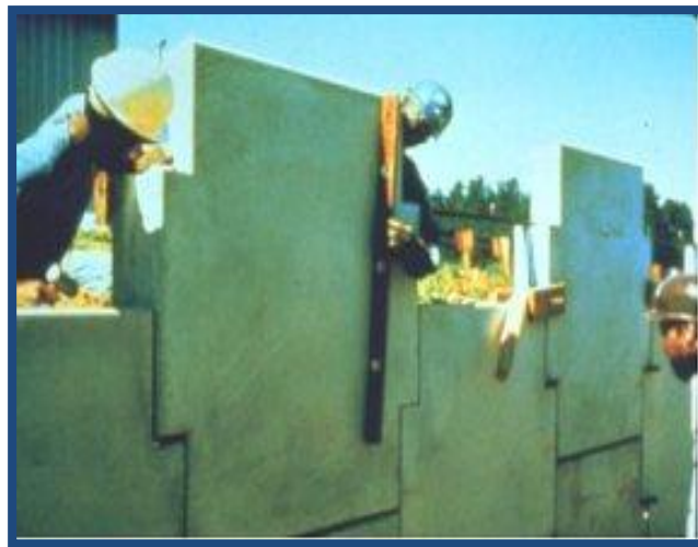
Figure 6-5: Checking Vertical Alignment
