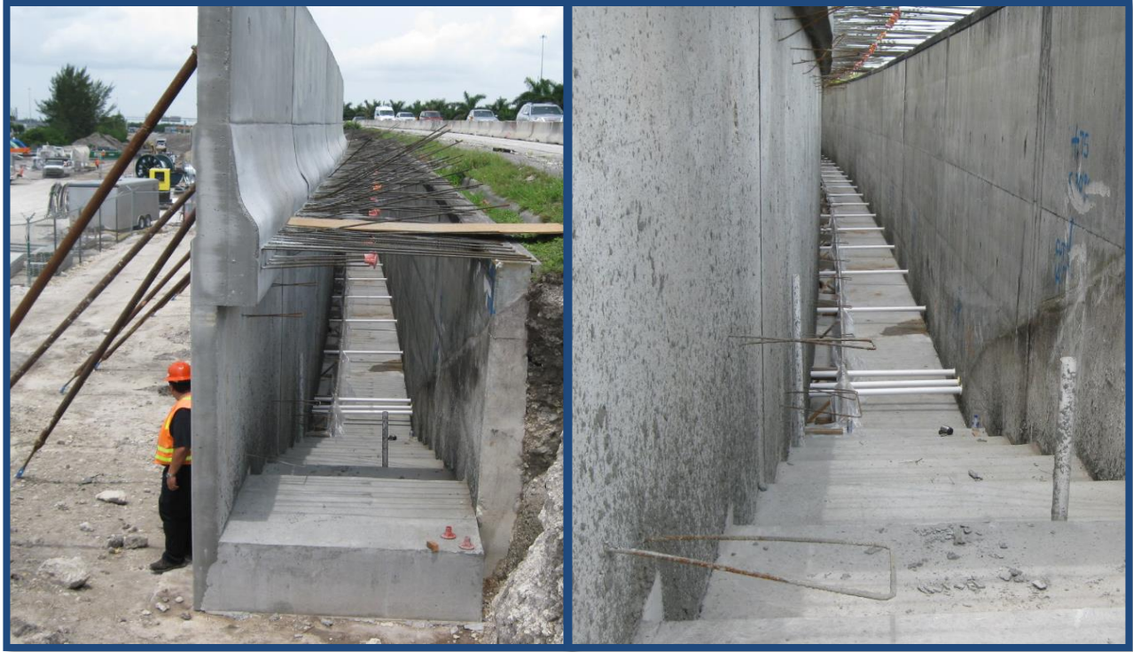
Figure 14-1: Cellular Concrete Wall
