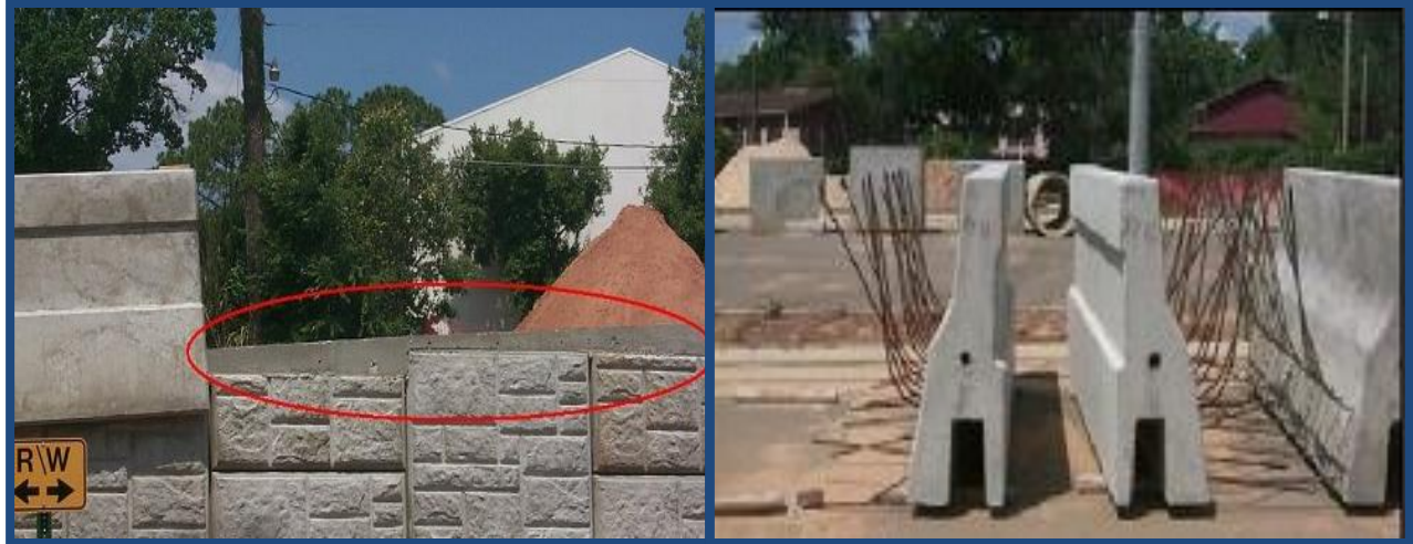
Figure 10-2: Precast Barrier (Leveling Concrete Indicated in Red)
