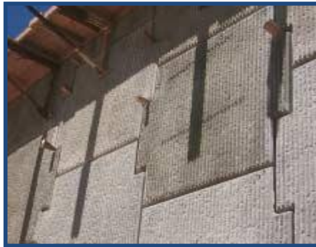
Figure 17-12: Wooden Wedges
