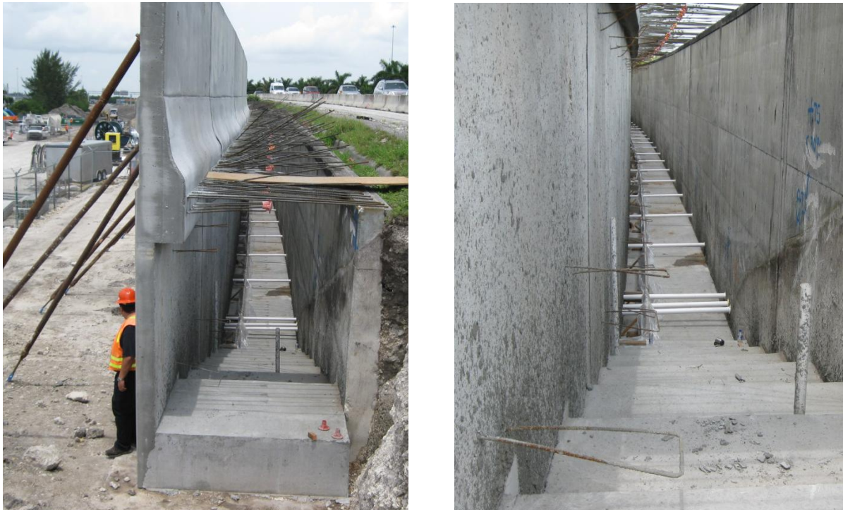
Figure 60, Cellular Concrete Wall
