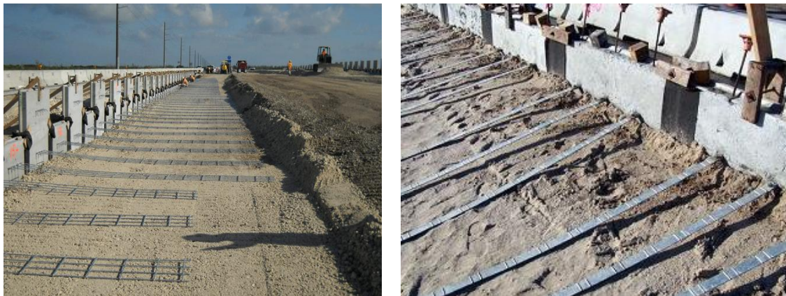
Figure 17 , Metallic Reinforcement (Inextensible). Left: metallic grid. Right: Ribbed Strips.
