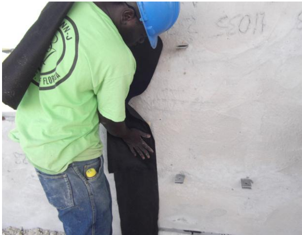
Figure 23, Filter Fabric installation
