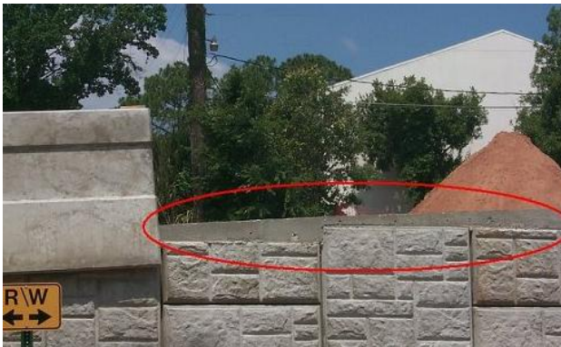
Figure 28, Precast Barrier. Indicated in red is the leveling concrete.
