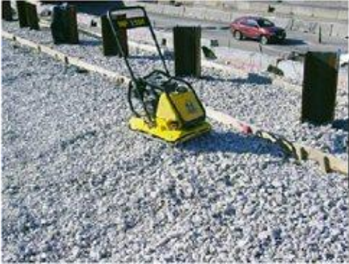
Figure 53, Typical compaction equipment used within 3 feet from the panel (must weigh less than 1000 lbs)
