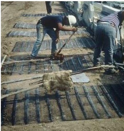
Figure 48, Tightening polymer Reinforcement
