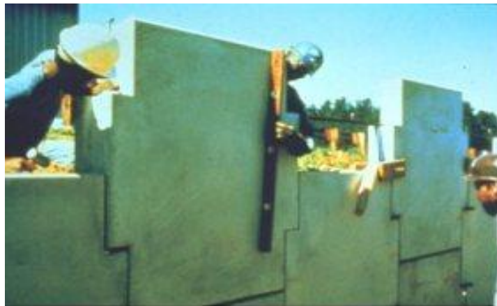
Figure 9, Checking vertical alignment
