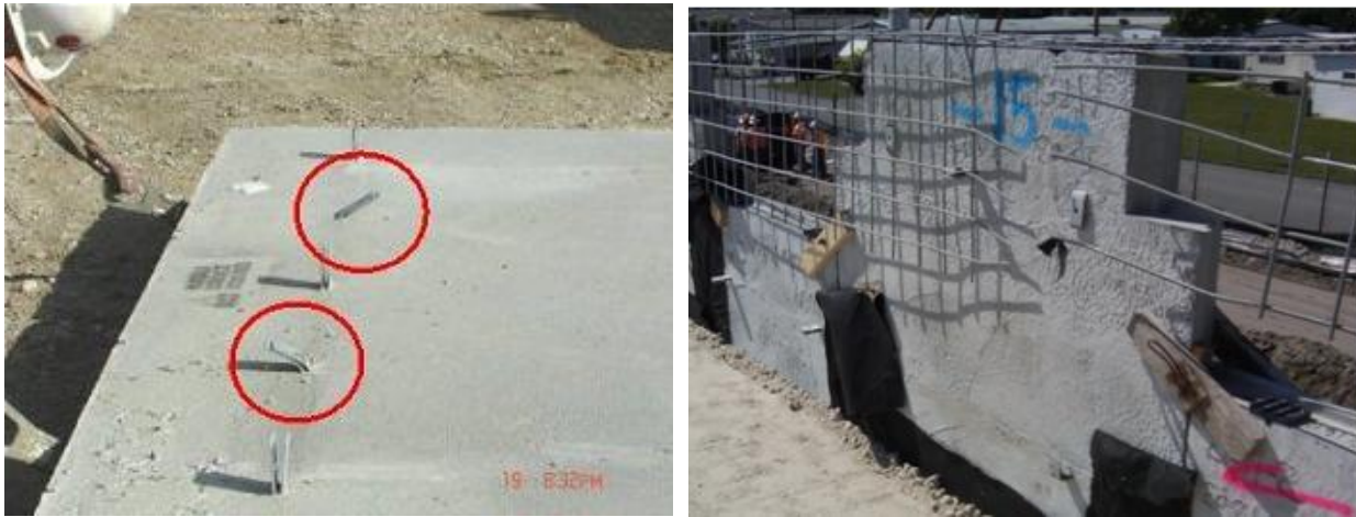
Figure 15, Damaged Tabs
