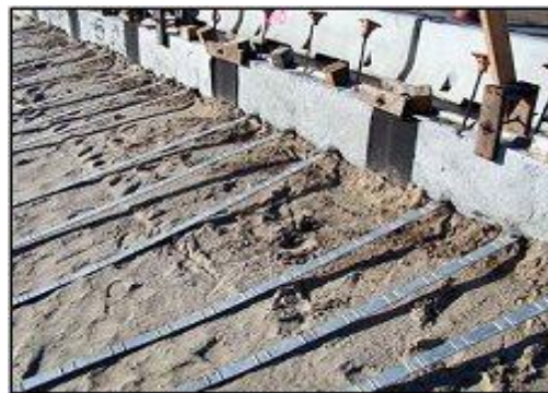
Figure 22, Reinforcement Connections
