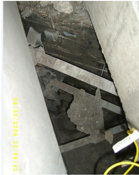
Figure 25, Loss of backfill through improperly constructed joint and filter fabric (Left: backfill washed through joint deposited next to the slip panel. Right: Void as observed from the top of wall)
