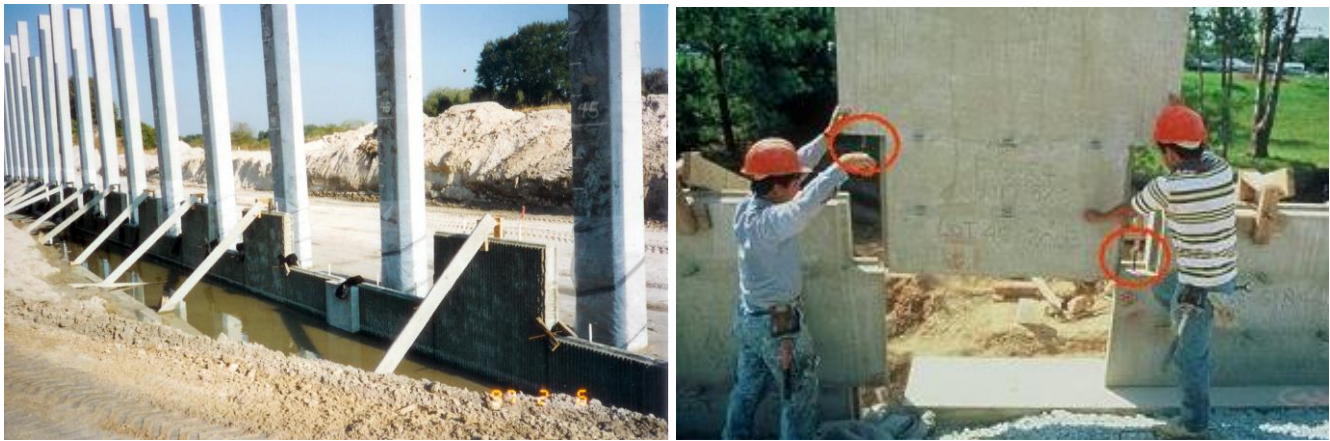
Figure 8, Placing and bracing Panels.
