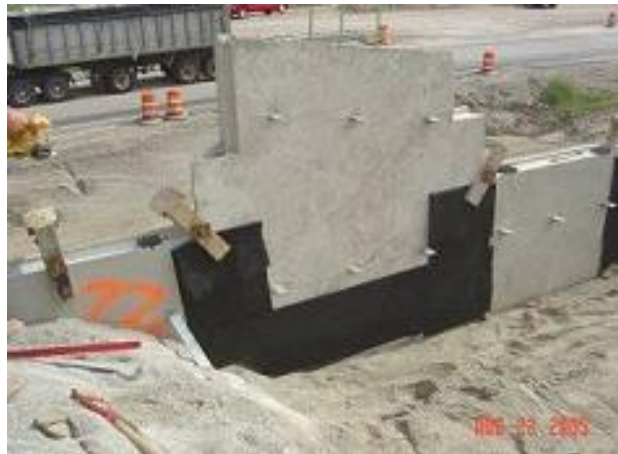
Fig 24, Filter Fabric installed at the joints
