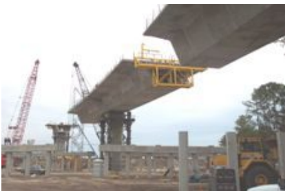
Segmental Bridge Construction for original I-595 airport bridges
