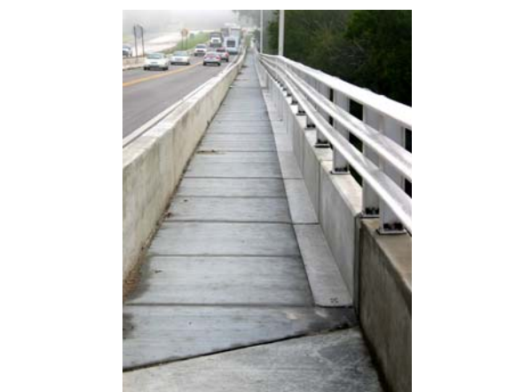
East End of Bridge Looking East
