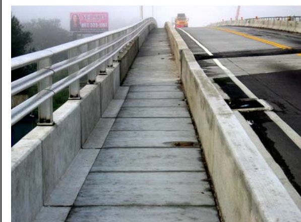
East End of Bridge Looking West
