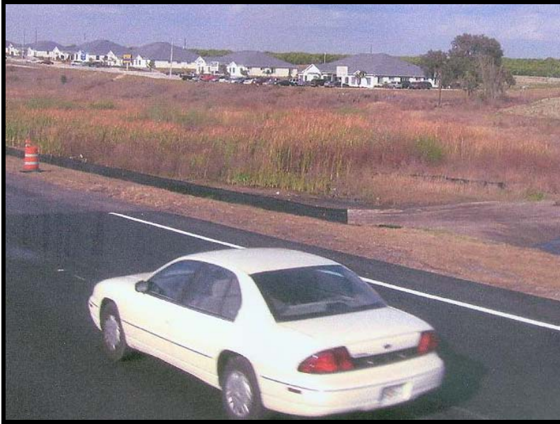
February 23, 2006 photo showing completed Friction Course
