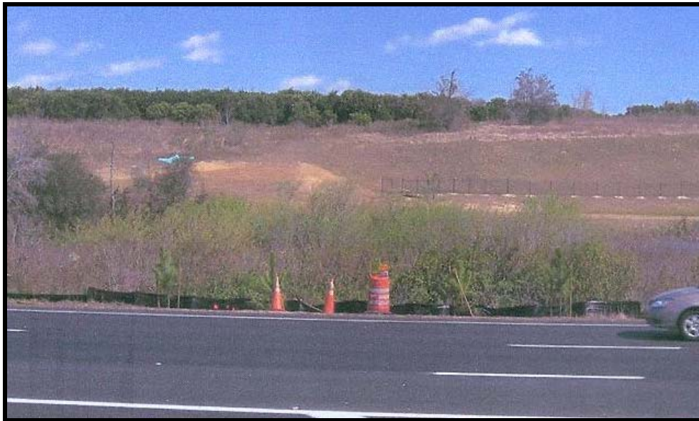
February 9, 2006 photo that shows Pond 4 with missing sod and fencing.
