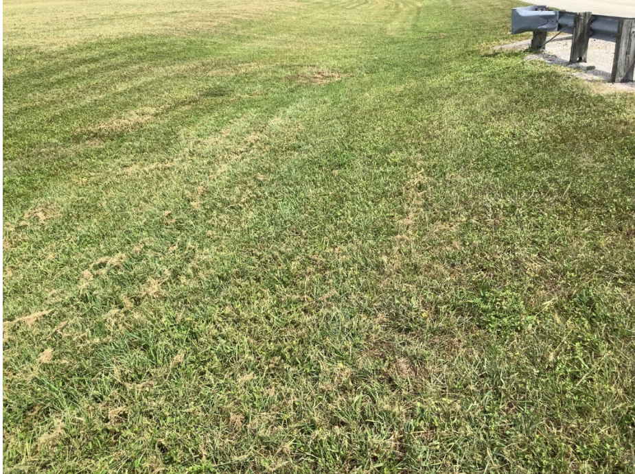
Figure 701-3 Well Maintained and Functioning Dry Swale
