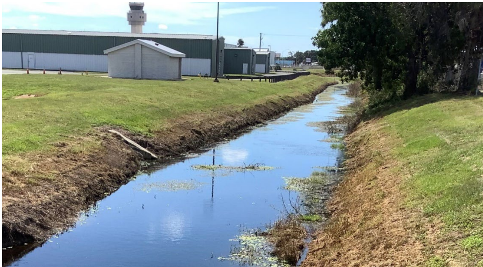
Figure 605-7 Steep-Sided Wet Swale
