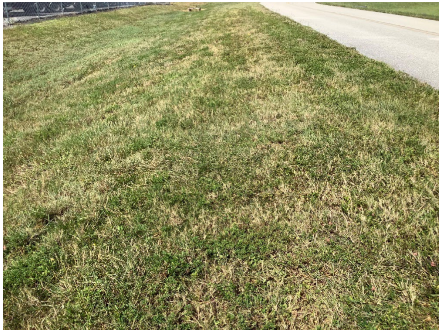
Figure 605-5 Typical Well-Maintained and Functioning Dry Swale
