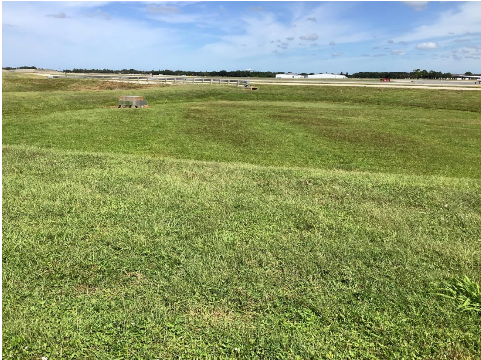
Figure 701-6 Well Maintained and Functioning Dry Retention Area
