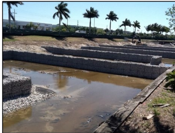
Figure J-4 Naples Pond Gabions Under Construction
