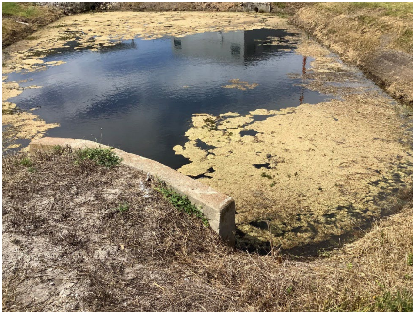
Figure 701-2 Algal Build Up and Bloom Requiring Maintenance
