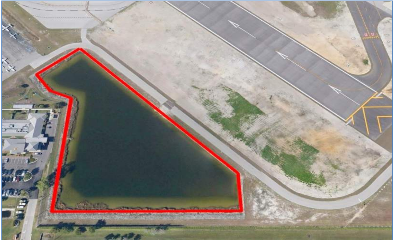
Figure 2 - Pond 214 Before It Was Modified
