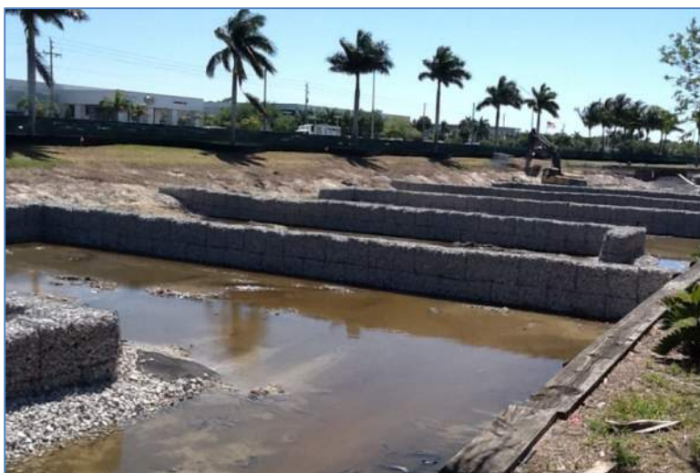
Figure 5 - Gabion Baffles Under Construction
