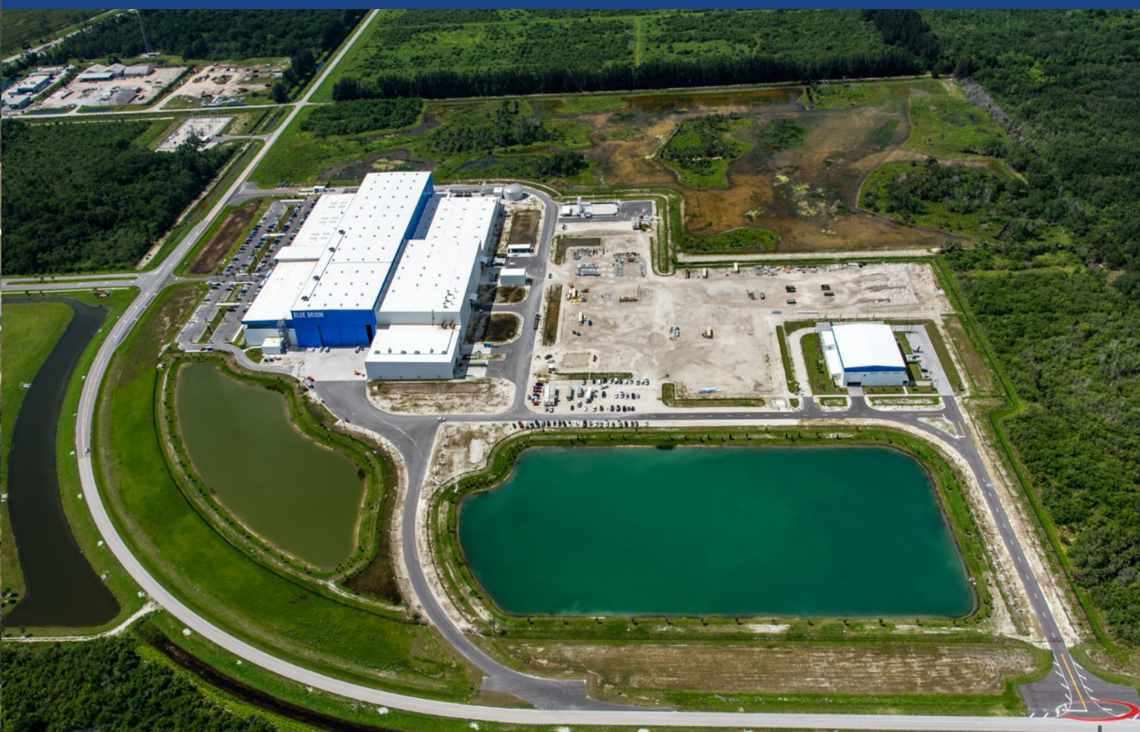
Blue Origin Manufacturing Complex (Under Construction)
