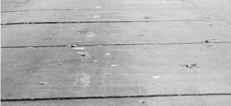
▲ Faulting of joints. Aggravated by heavy traffic in one direction. Could improve surface by grinding.
