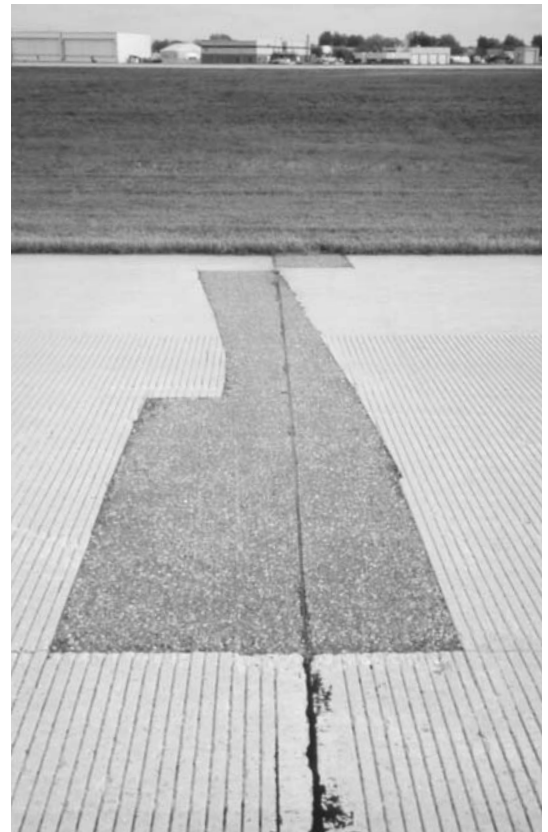
▲ Full depth joint repair. Very good condition.
