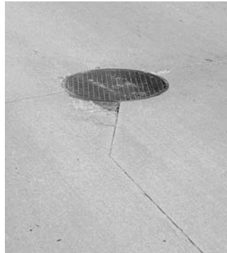
▲ Isolated spall at manhole.
