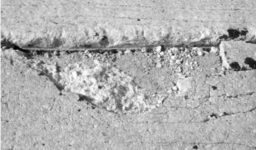
▲ Failed joint with severe spalling and pothole.
