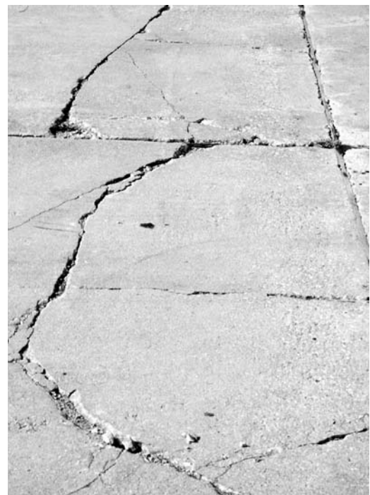
◀ Closely spaced, hair-line, transverse cracks indicate slab is broken and needs replacing.
