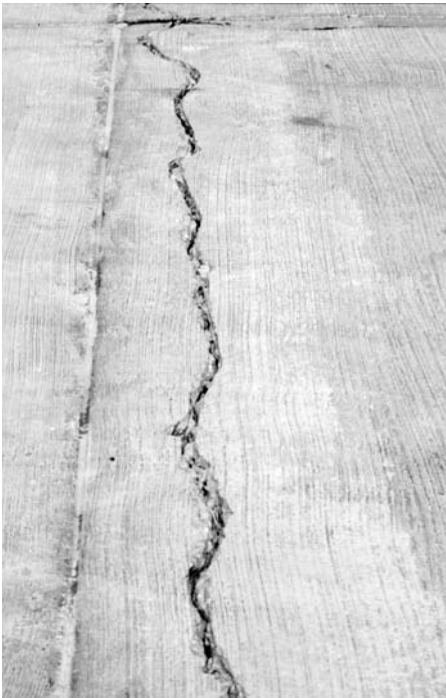
▲ Hairline slab crack. Tight with no spalling.
