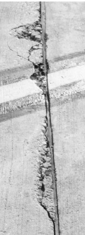
◀ Spalling along a joint.
