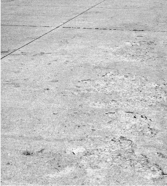
▲ Isolated spall at manhole.
