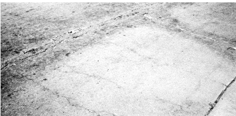
◀ Closely spaced, hair-line, transverse cracks indicate slab is broken and needs replacing.
