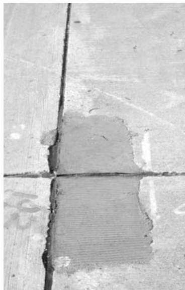
▶ Joint repair with asphalt. Very good condition.
