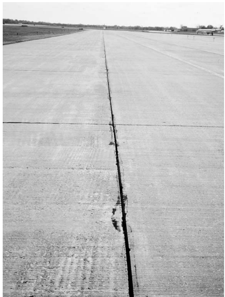
▲ Joint sealant deterioration on apron. Slab is in good condition.
