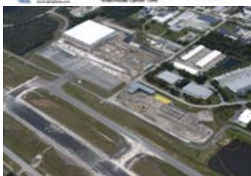
Photo courtesy: Lakeland Linder International Airport
