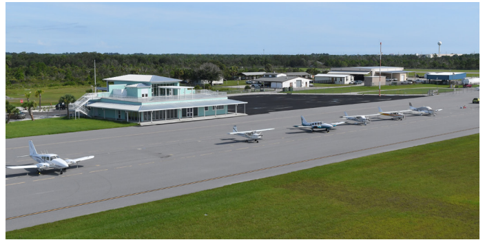
Photo courtesy: Valkaria Airport
