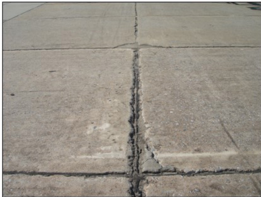
Joint Seal Damage
