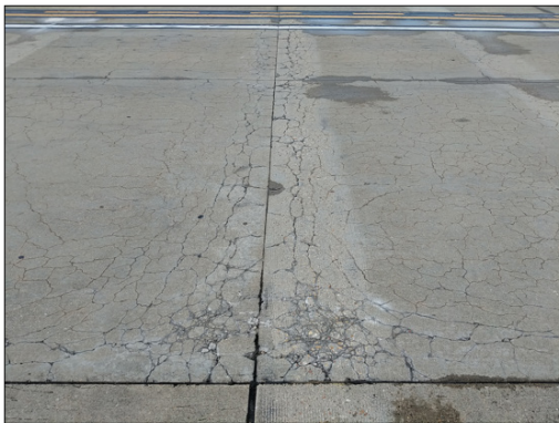
Alkali Silica Reaction (ASR)
