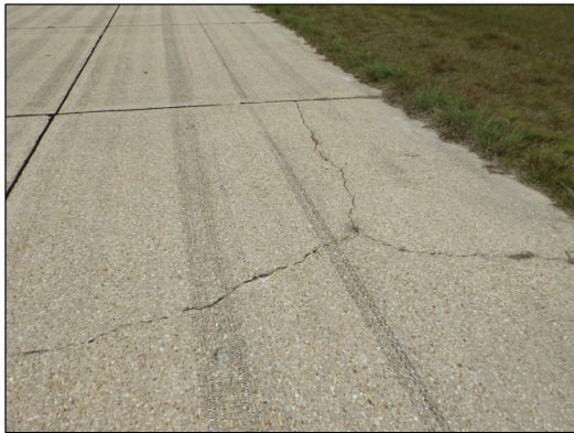
LTD Cracking
