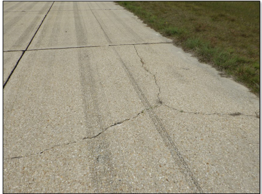
LTD Cracking
