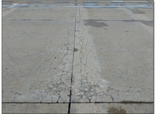
Alkali Silica Reaction (ASR)
