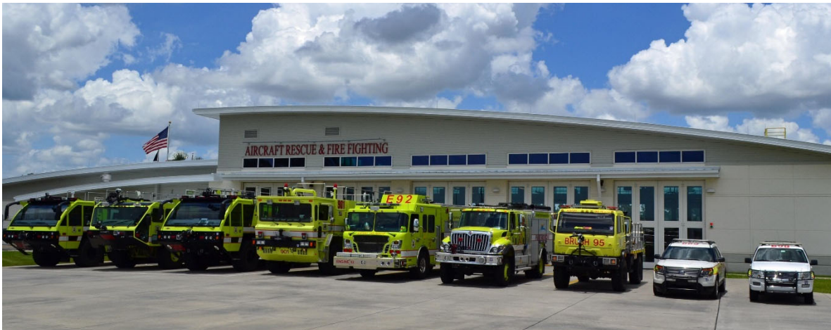
Figure 16 – On-Site Aircraft Rescue Firefighting (ARFF) Facilities
