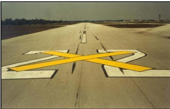
The yellow cross shows that Runway 22 is temporarily closed.
