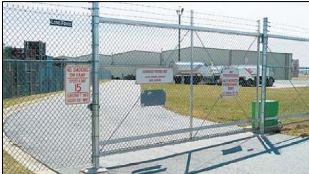
A typical security gate on airfield
