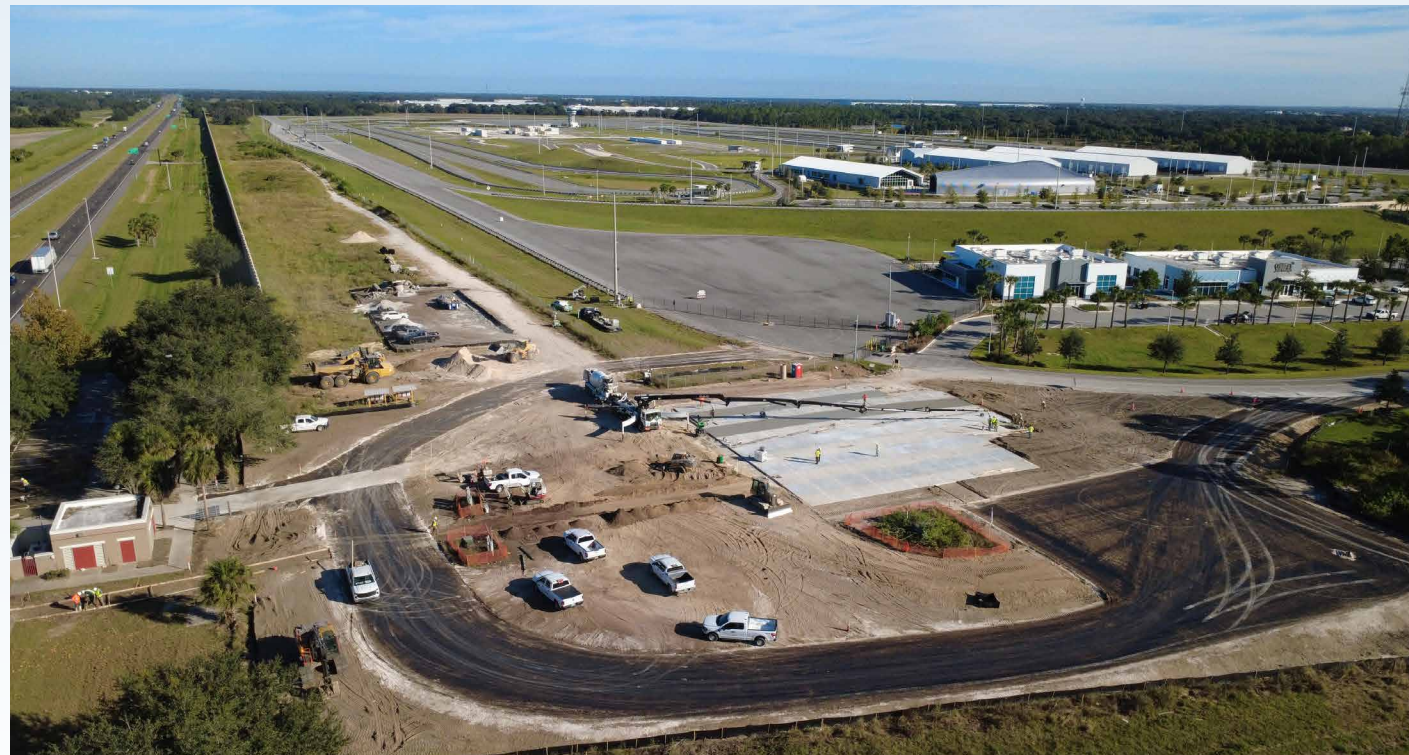
SunTrax Air Phase 1A Under Construction - Complete week of November 3, 2025
