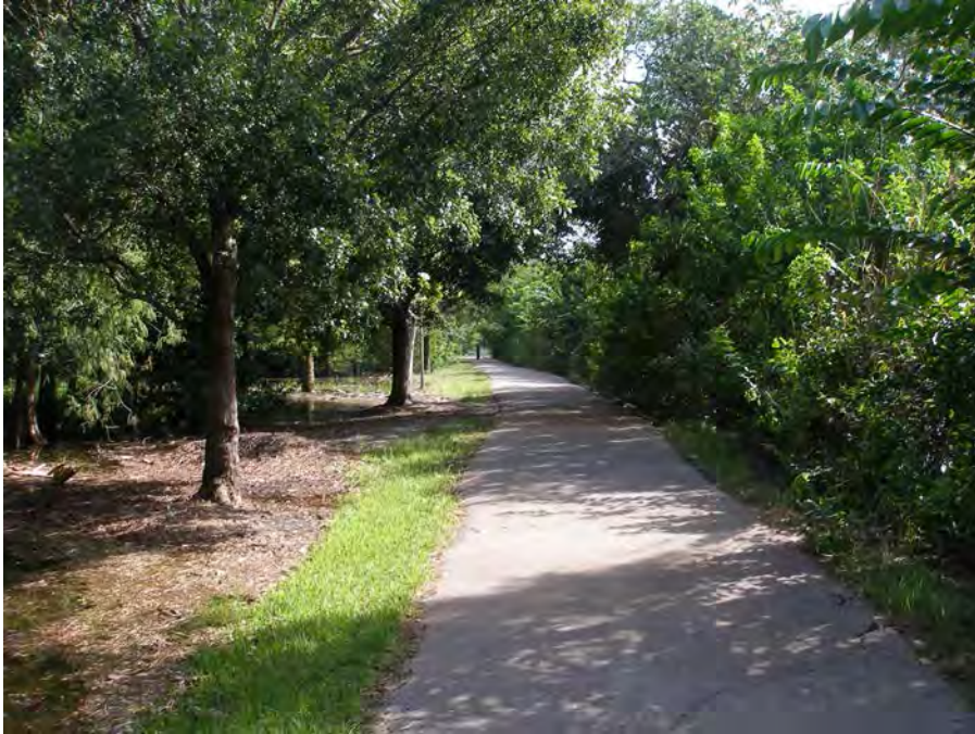
Photo 3: Stan Goldman Park, existing trail between Hollywood Boulevard and Johnson Street, looking north (typical). Note all other facilities associated with Stan Goldman Park are at the north end closer to Johnson Street.
