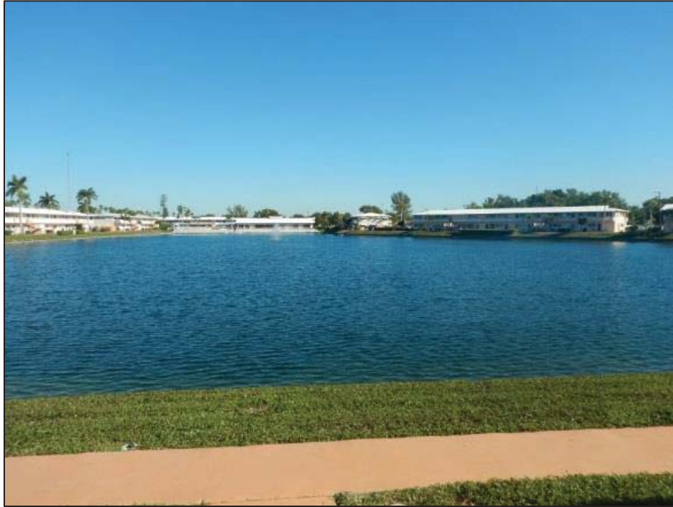
Photo 7: OSW-2 – Stormwater retention pond within Ro-Len Lakes Gardens (typical).
