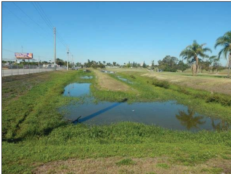
Photo 12: OSW-7 – Stormwater retention area within the Orangebrook Golf and Country Club.
