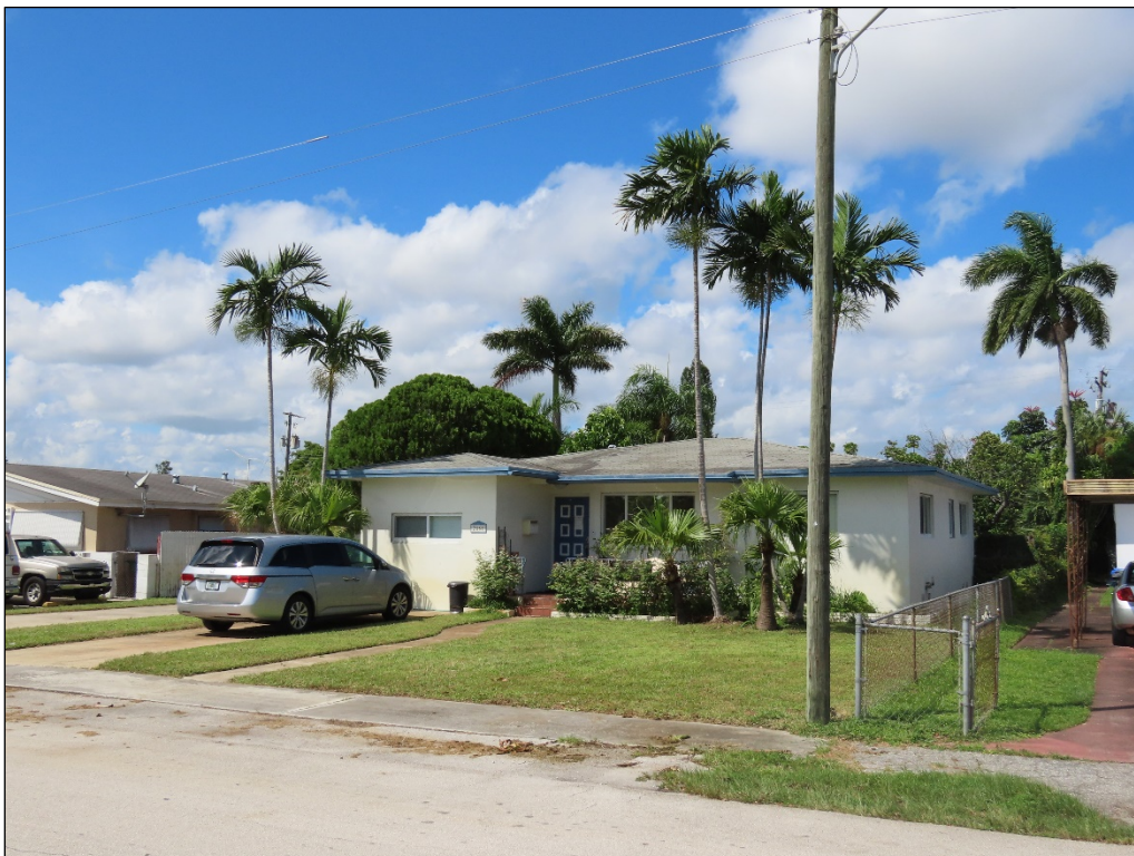
Figure 10.11 – 2851 Polk Street (8BD7711), c. 1956, considered National Register- ineligible, facing Northwest
