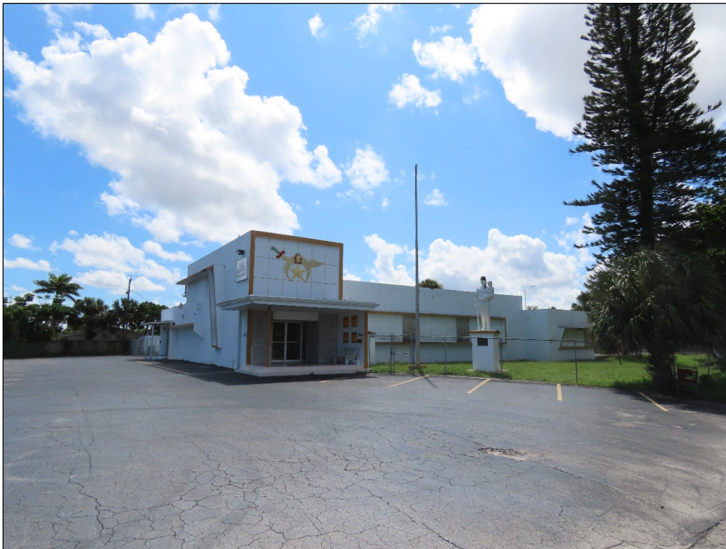
Figure 10.13 – Broward (f.k.a. Hollywood) Shrine Club, c. 1959, considered National Register-ineligible, facing Southwest
