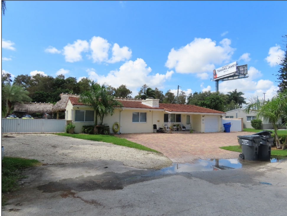
Figure 10.15 – 800 N 29 th Avenue (8BD7714), c. 1954, considered National Register-ineligible, facing Northwest
