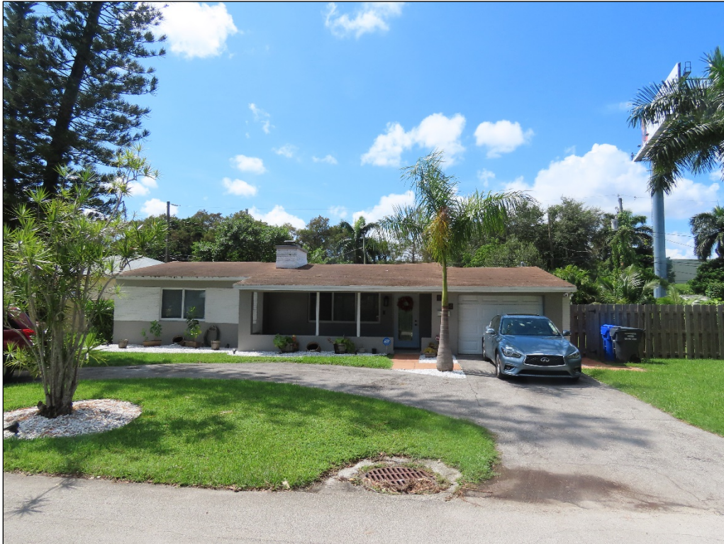
Figure 10.16 – 804 N 29 th Avenue (8BD7715), c. 1954, considered National Register-ineligible, facing Northwest
