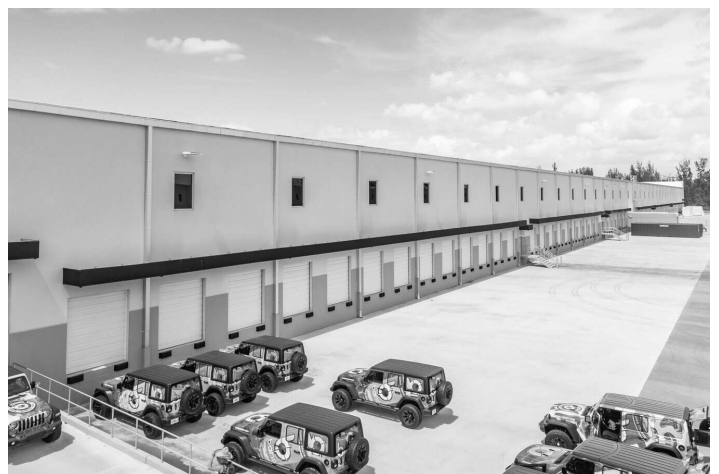
Rear Dock Doors
