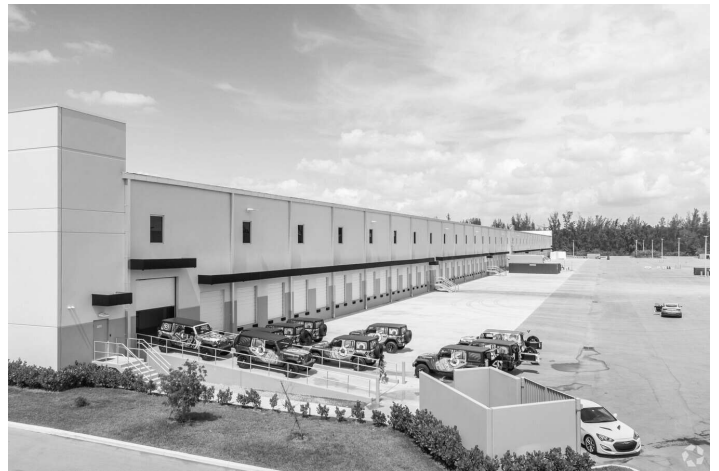
Rear Loading Bay
